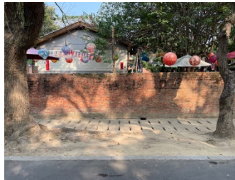
Figure 4: Exterior wall of residence
