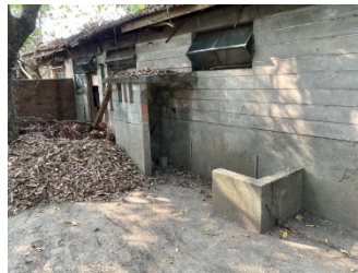
Figure 6: Space for the old water heater behind the residence
