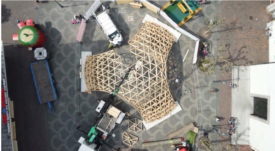
Figure 1. A 15m span research demonstrator: ReciproFrame timber gridshell
