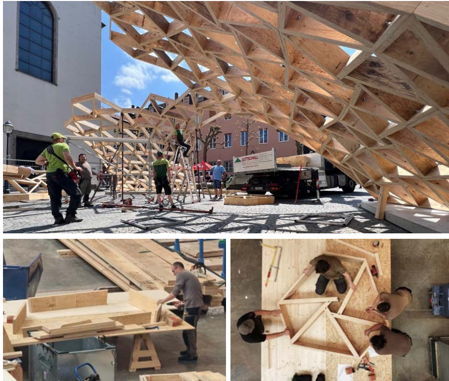
Figure 4. Indoor and onsite assembly of beams and cassettes
