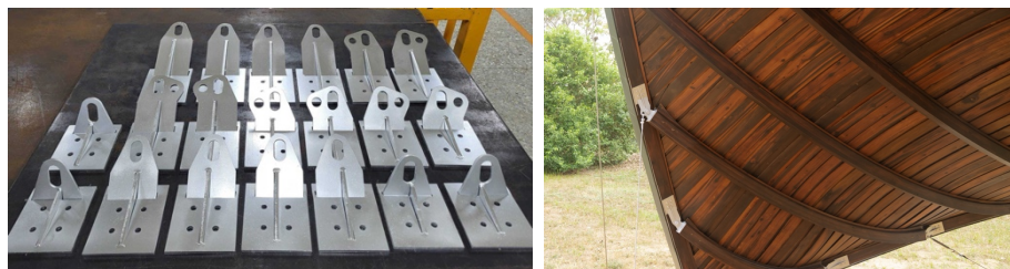
Figure 9. a) Prefabricated steel connectors, b) Installed steel connectors
