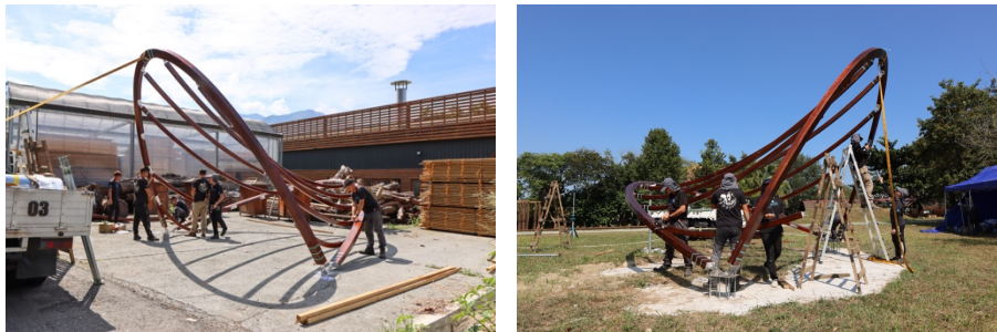
Figure 10. a) Mock assembly, b) Onsite assembly
