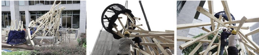
Figure 10. The assembly process of the fabric and the wooden structure
